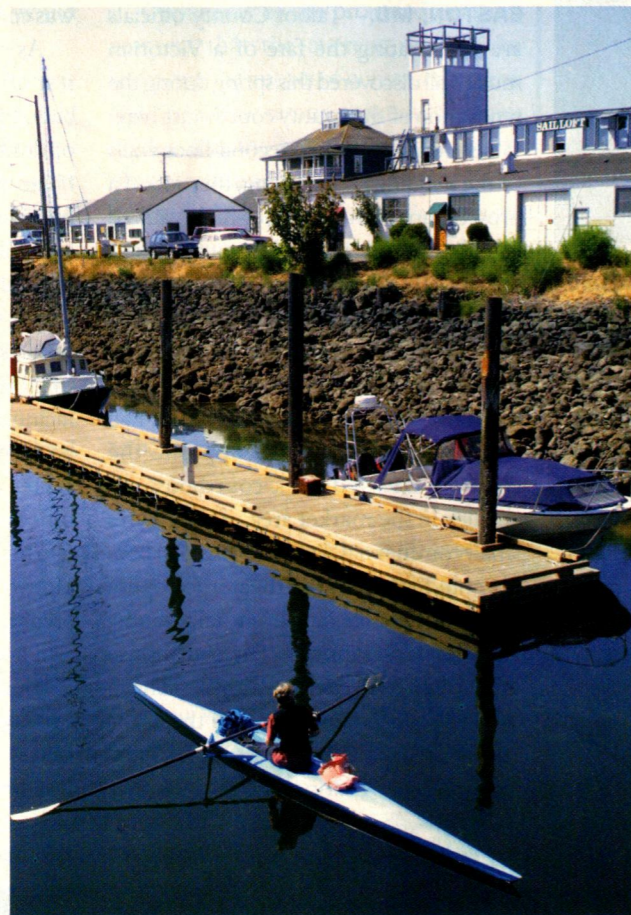
A kayaker, above, and strollers, opposite, take in the utilitarian if run-down assets of Point Hudson.
